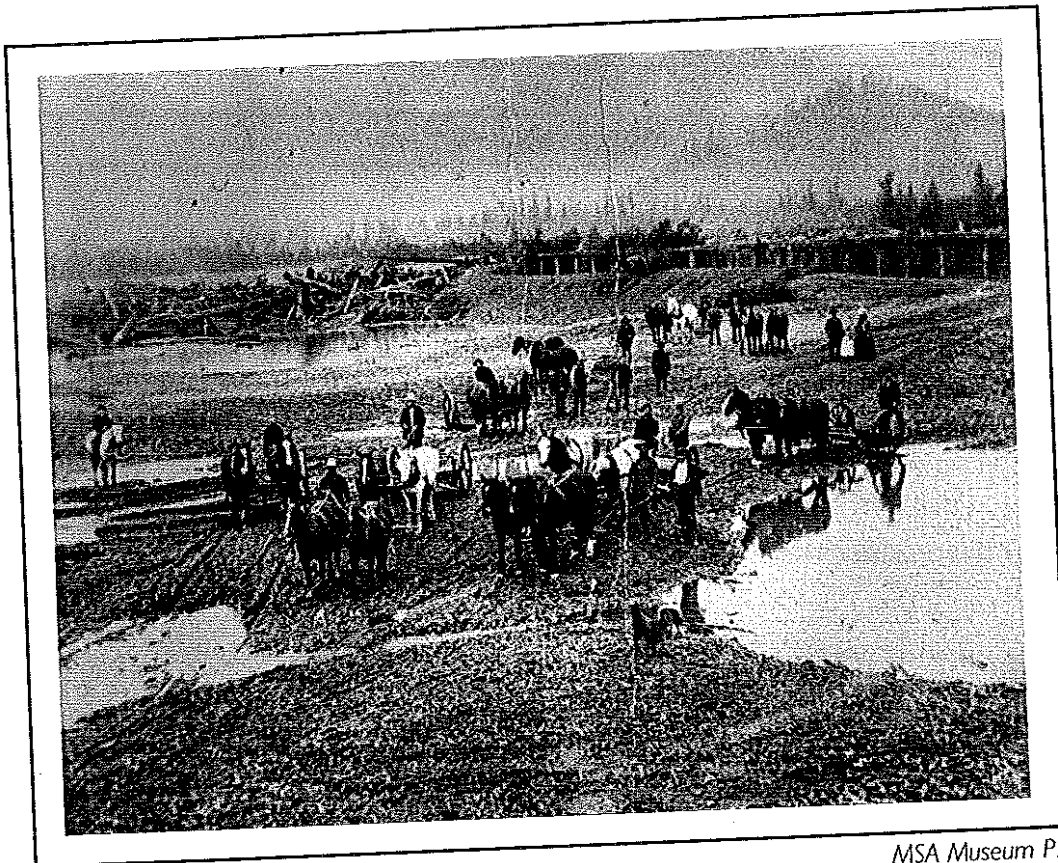
The drainage project begins.
